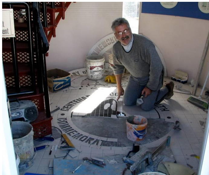
Pictured: Tiler Allan Mallard creating the mosaic masterpiece on the Lighthouse floor.
