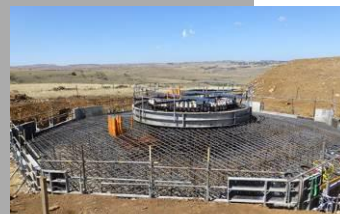
TOWER BASE AT BOCO ROCK
