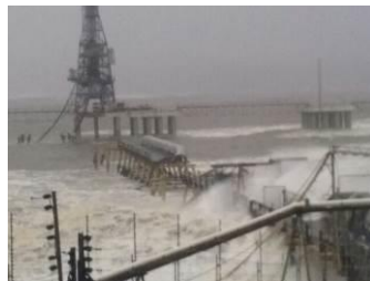
Waves destroy the chip mill wharf and conveyor
