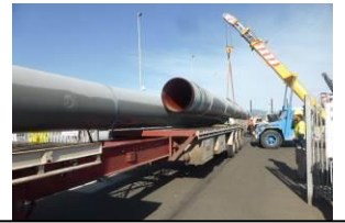
20 meter long gas piping to be used to repair the chip mill jetty is unloaded at the breakwater wharf in Eden – Rob Whiter
