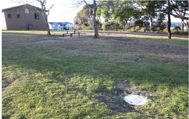
The probable hydrant from which the Premier released water that heralded the piped system for the town, in 1956.
